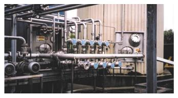
The site has its own two bore holes that can produce all their water requirements, but can also connect onto mains water if required. Water is an essential commodity at the dairy and is used for a host of water services such as wash downs, cooling etc. The water is softened before use to avoid leaving any residue on the production surfaces.
